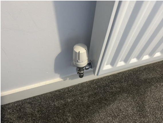
R5-22 | Radiator thermostatic valve and adjacent floor Photographed 21 August 2026 at 15:36
