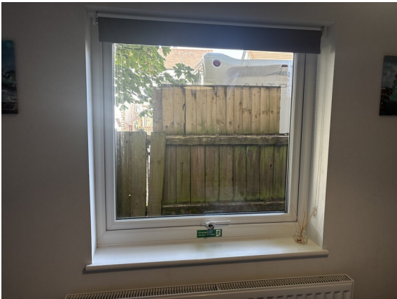
R5-20 | Window, blind and sill Photographed 21 August 2026 at 15:36
