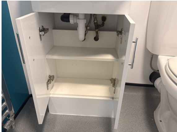
ES-05 | Vanity unit - doors open and interior Photographed 21 August 2026 at 15:40
