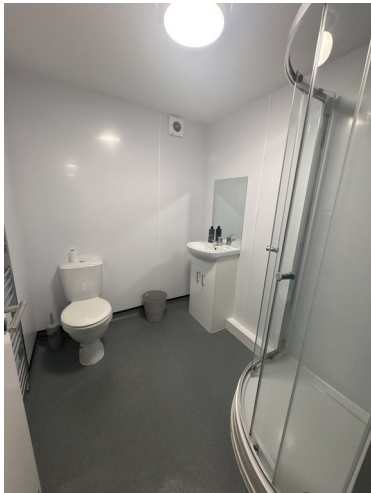
CA03 | Communal bathroom - ceiling and upper-level overview Photographed 21 August 2026 at 15:21
